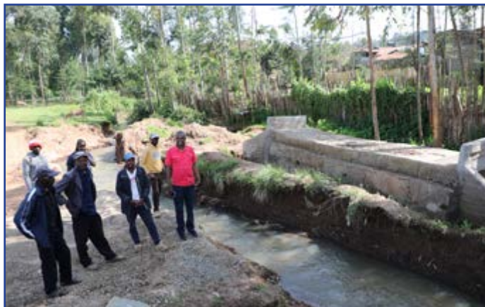
Hon. Ngware interacts with residents of Molo during a site visit to the ongoing construction of the Munyu-Upendo Bridge
