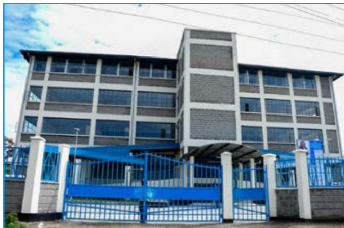
Front view of the new Bondeni Modern Market
