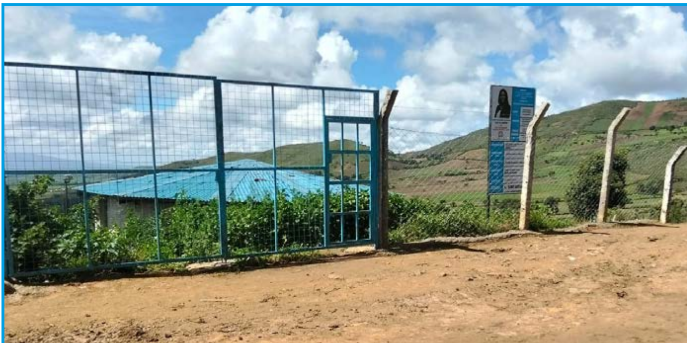
Fencing and Solarization Works at Nkampani Water Project, Maiella Ward
