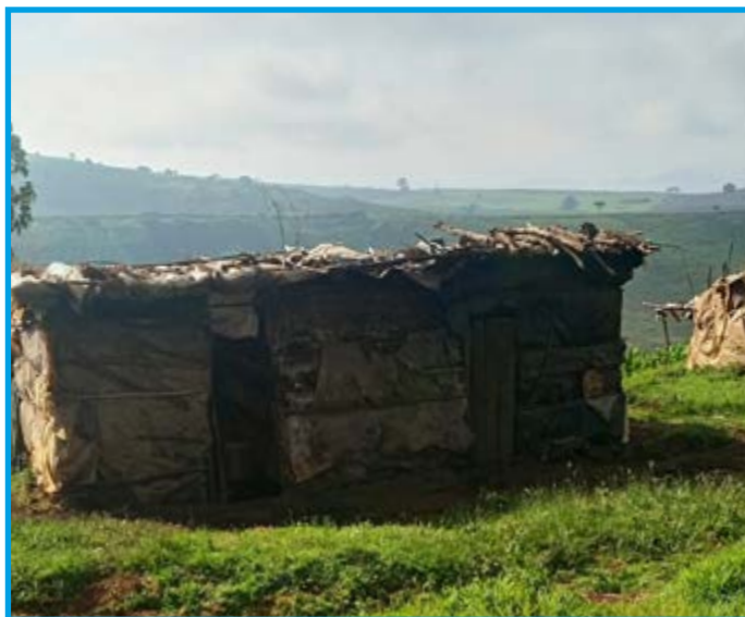
Destroyed homes in Maiella Ward, Naivasha, following a land dispute
