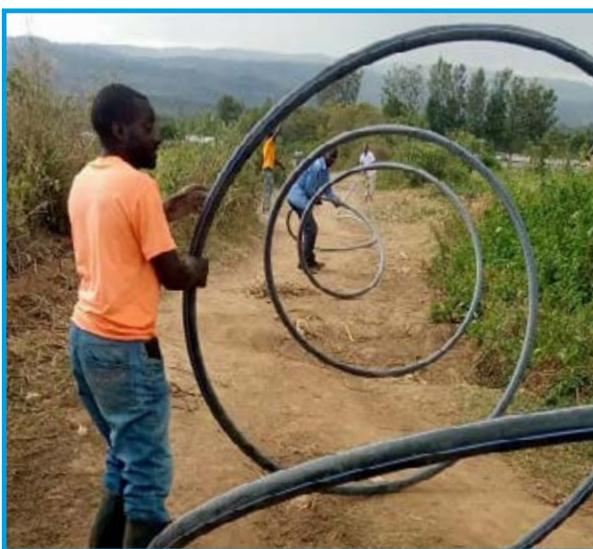
Water pipeline installation to individual homesteads in Kipkonyo, Maiella Ward
