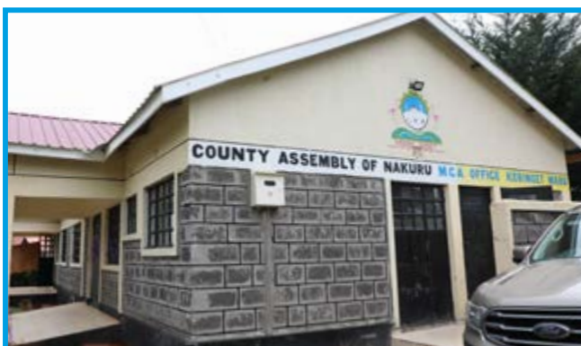
Main block, Keringet Ward office
