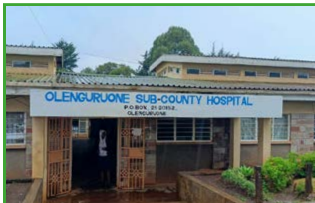
Olenguruone Sub-County Hospital
